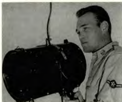
Light guns are used now only to clear planes when radio failure occurs and to control the movement of vehicular traffic on the airport.
