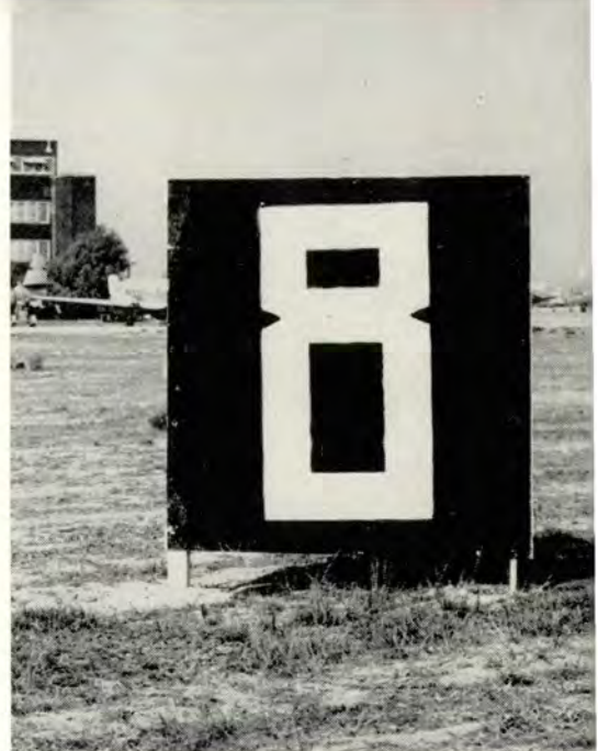
Runway distance markers are designed to check aircraft performance during takeoff.
